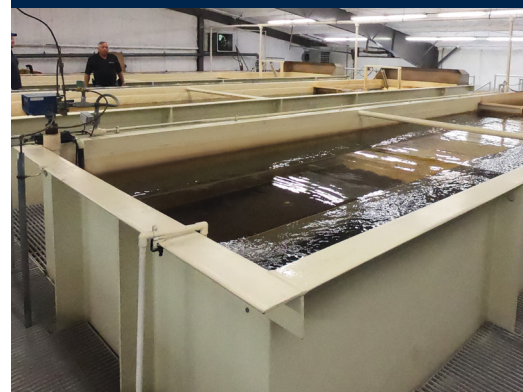
Filter bed media was installed atop the new in-bed air grid for air-water backwashing.
