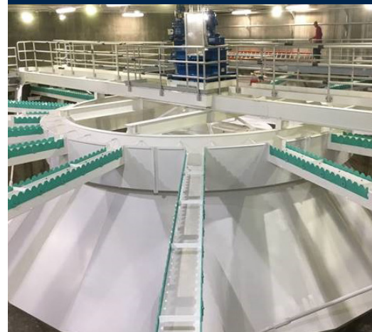
Solids CONTACT CLARIFIER under Construction
