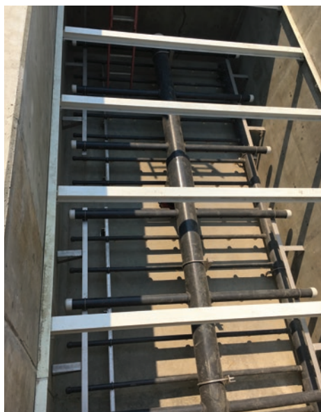
Raw water distribution piping in Adsorption Clarifier cell
