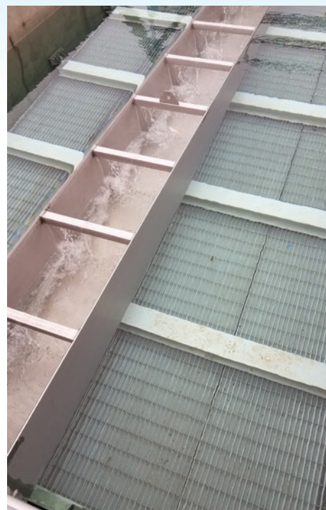
An Adsorption Clarifier unit in production at Miners Ranch
