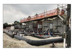
The mobile clarifier unit can handle a total suspended solids (TSS) load of up to 6,000 mg/L with integral sludge pumps that are already piped, wired, and ready for service.
