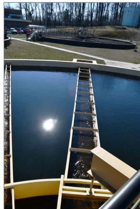
New and retrofit CONTRAFLO units on-site at the City of Lebanon Authority WTP
