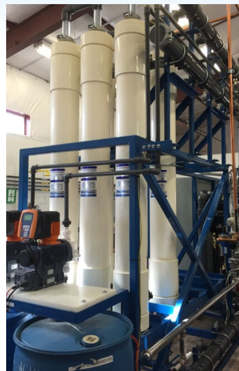
Only half the ultrafiltration racks are populated due to current demand. The capacity of the system can be doubled quickly and inexpensively by installing additional modules. All system components are sized for the increased capacity to limit costs associated with expanding the system.
