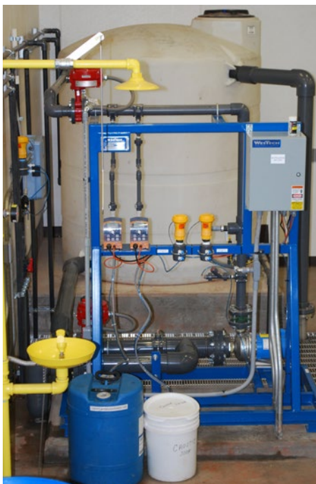
An optional neutralization system was included with this equipment to allow for discharge of chemical solutions used during membrane cleaning.
