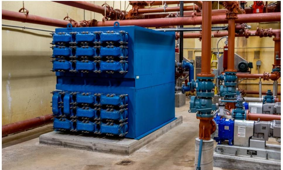
*Tube-in-tube heat exchanger*
