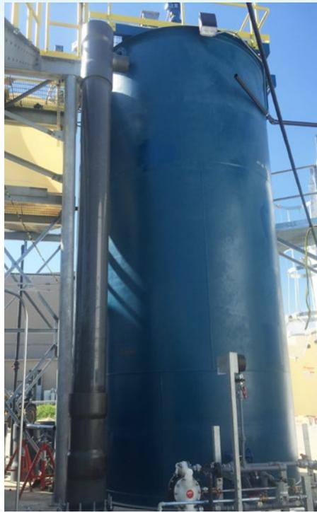
reaction tank 1 where lime addition was used to adjust pH. Water flowed via gravity through two more reaction tanks where ferric chloride and organosulfide were added to precipitate the metal hydroxides. In addition, polymer was added for flocculation. From there, the water was sent to a clarifier to settle and remove solids.
