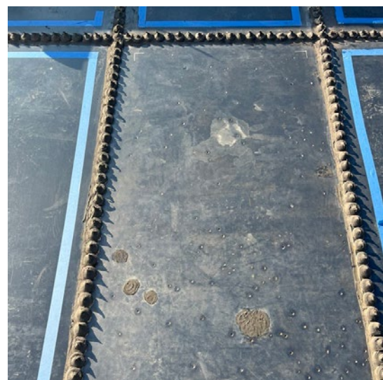
Close-up view of the corrosion on the panels inside the tank.
