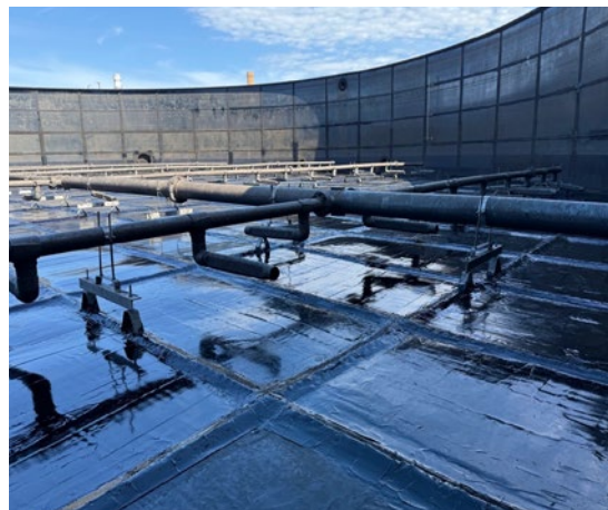
View from inside tanks after application of Chevron Industrial Membrane (CIM) elastomer-type epoxy is completed.
