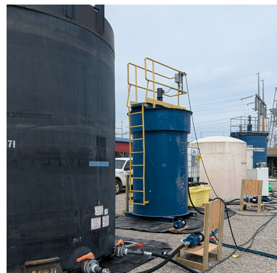
Pilot pre-treatment equipment included: thickener, reaction tanks, and clarifier shown here.
